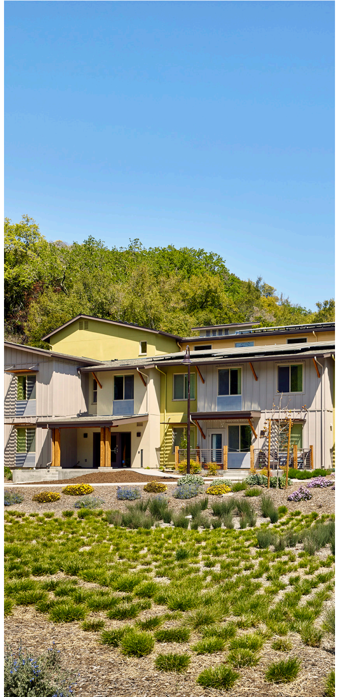
Our project in Marin County, a low income and formerly homeless senior housing development that was hard fought over for almost a decade, continued construction through the beginning of the pandemic, maintaining safety of the workers. Successfully completed, it welcomed its first residents in July of 2020 and served as a vaccination site for all the residents in the spring of 2021.
