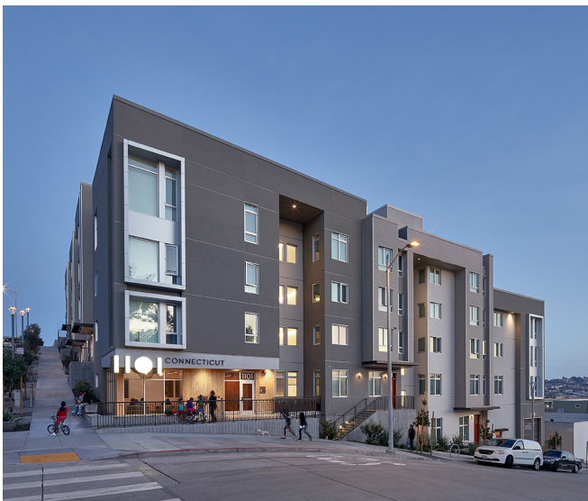
1101 Connecticut, San Francisco, CA: LEED Platinum - rooftop PV, solar thermal, 22k gal stormwater cistern, and 100% of stormwater treatment onsite.
